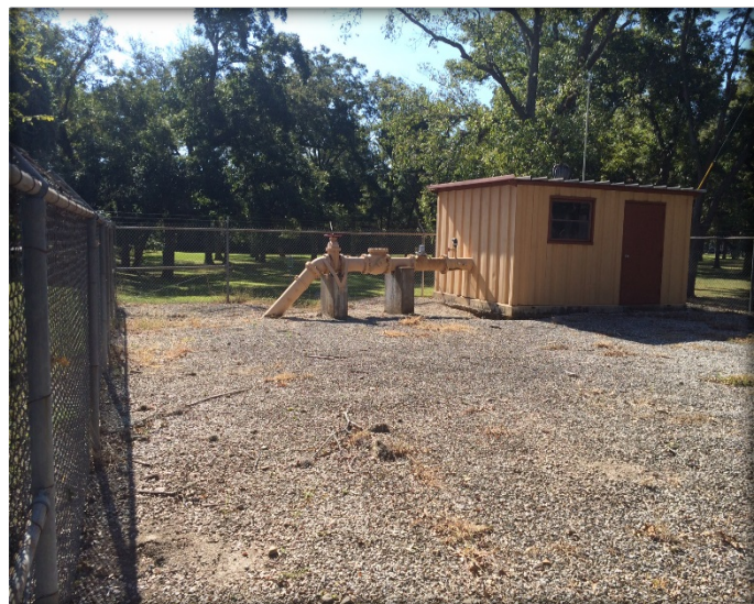
Figure 1: Existing Well 19 Pumphouse and Piping
